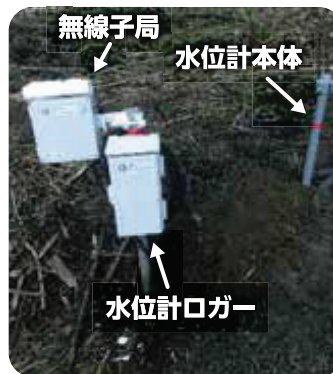
水位計 GENESIS/GWI (Ground Water Inspector)
